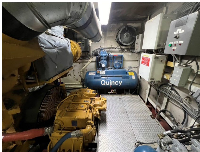
Figure 3: Ship Check Picture-Gearbox proximity to Frame 92
